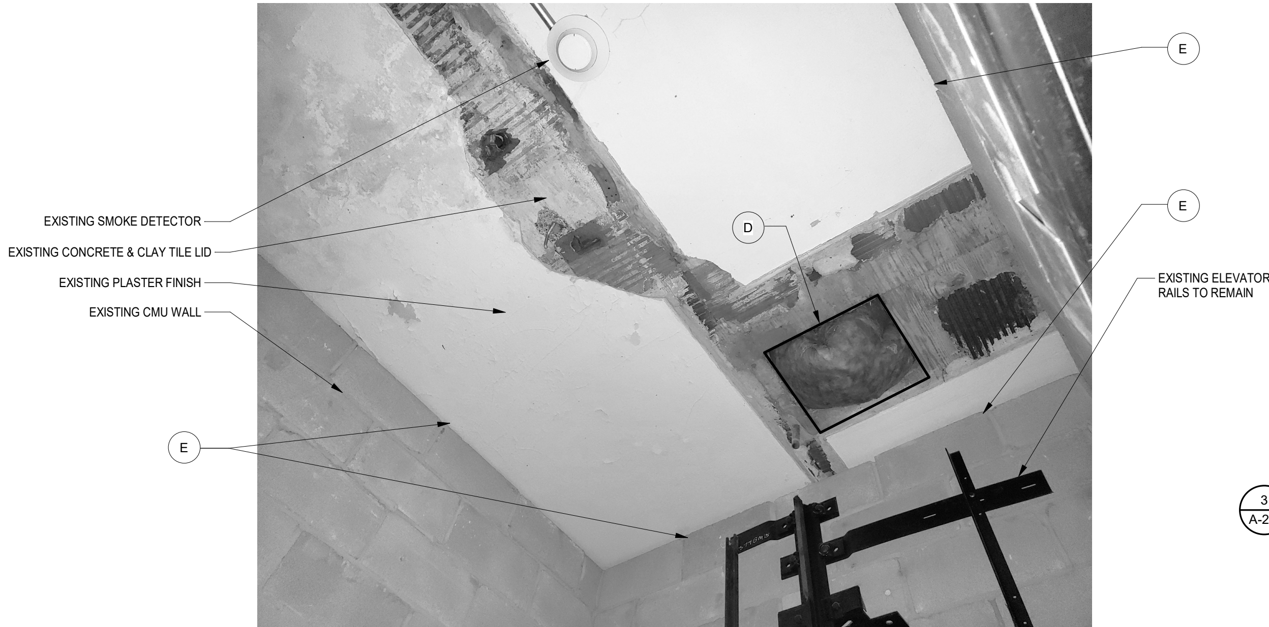
PHOTO 1: CEILING OF ELEVATOR SHAFT.
