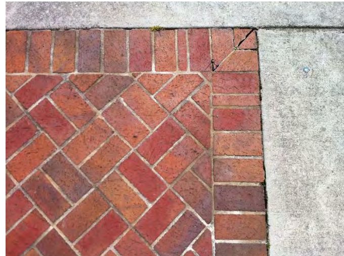
Mortared Clay Paver Field and Banding
