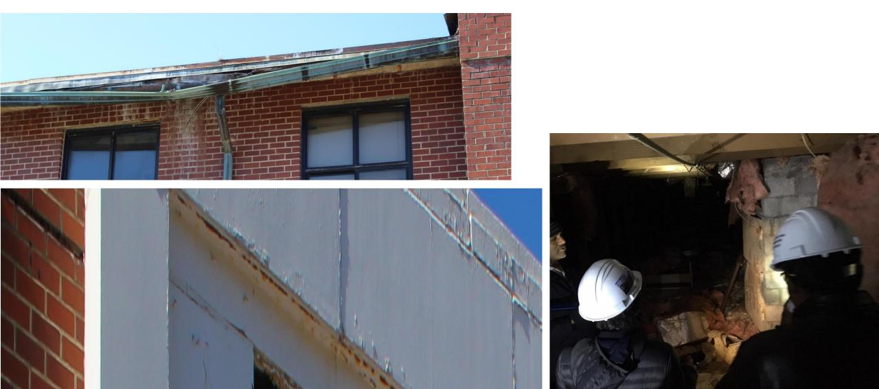
The photo on the left shows extensive paint chipping and mold growth on due to the exterior decline of the building envelope. The photo on the right shows the foundation of the building that is the same as Grayson and Walker Wood, but also show the levelness of the ground. This aspect allows for a future uses at minimal cost.
