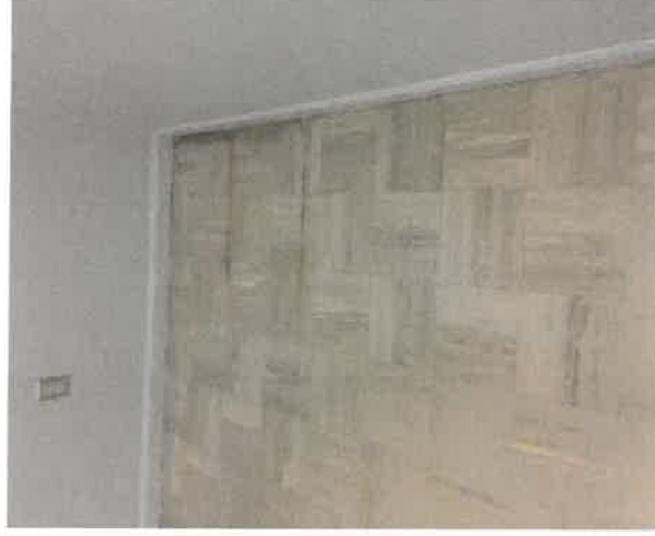
Carver Complex north wing VAT flooring.
